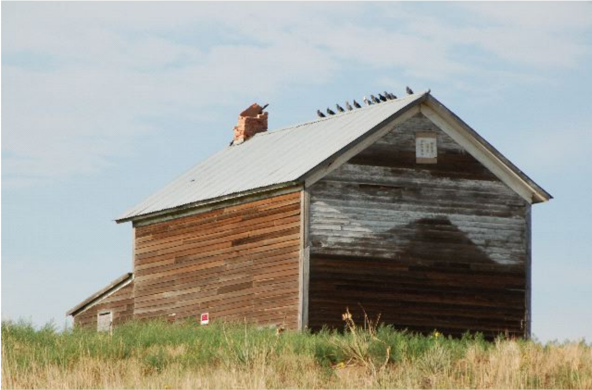
Abandoned School House, Emmons County – North Dakota
